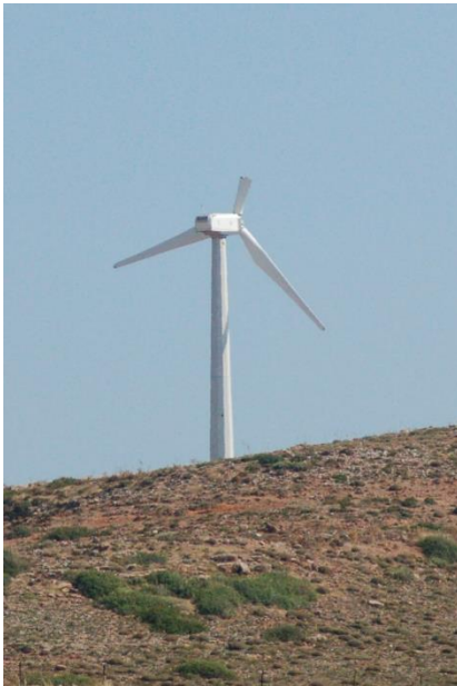
Figure 8. Damaged turbine at Crete, Greece
